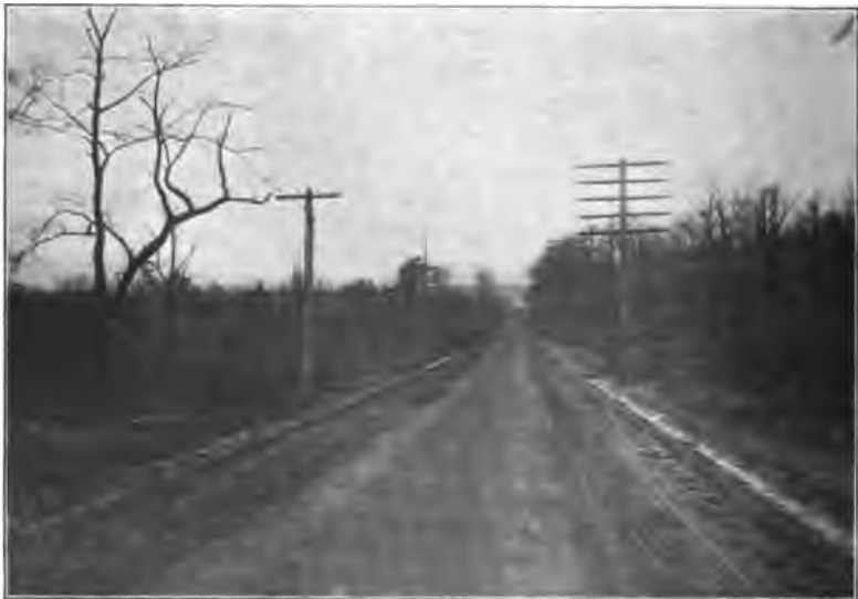
Navesink road, near Stone Church, Monmouth Co., after completion.
